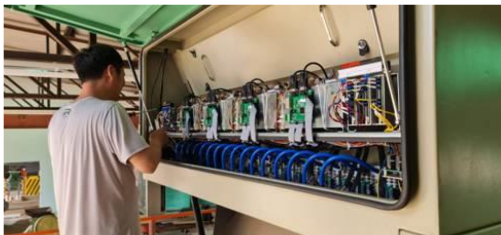
Figure 2. Angelon technical expert busy with the commissioning of the optical sorter.
