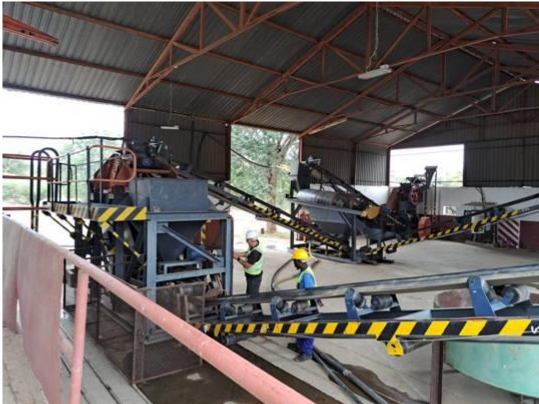
Figure 1. The commissioning of the processing plant in progress.
