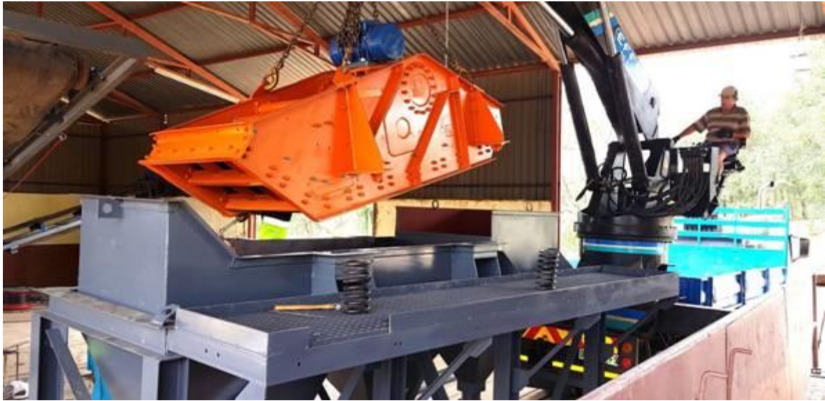
Figure 3. Installation of the dewatering screen.
