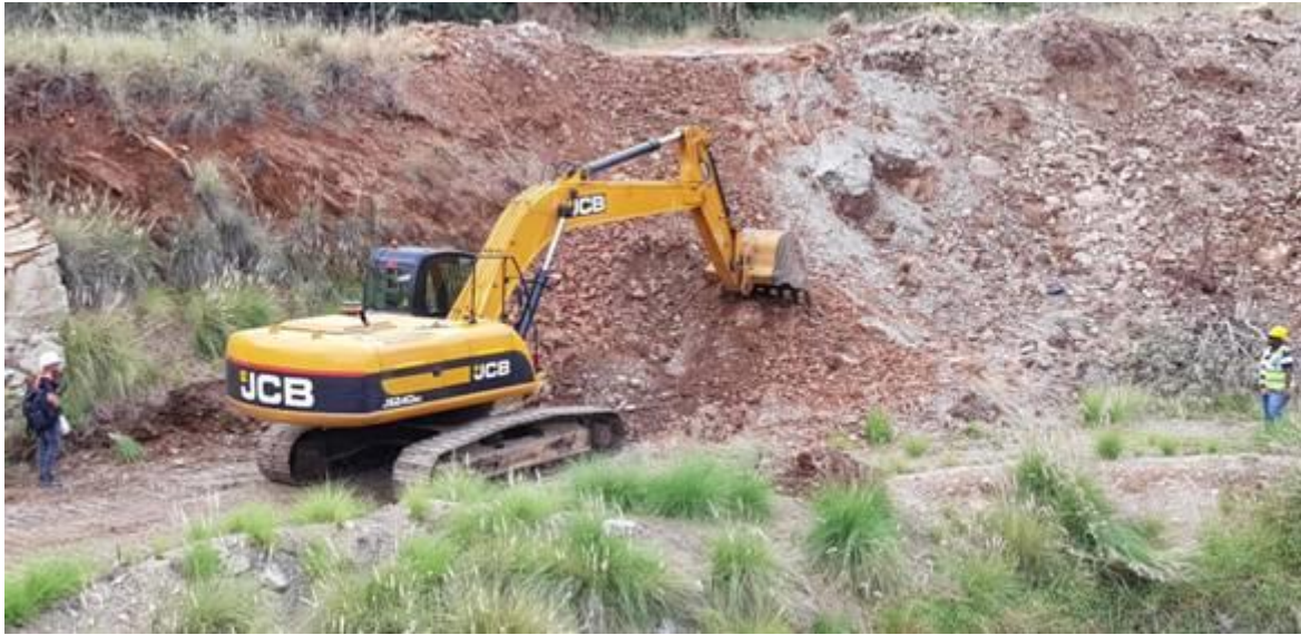
Figure 1. On site road construction in progress
