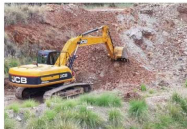
↑ A 24-tonne excavator working in one of the Gravelotte pits
